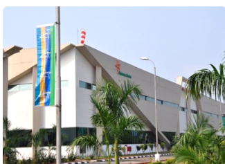
Pharmaceutical Facility Baddi, Himachal Pradesh
